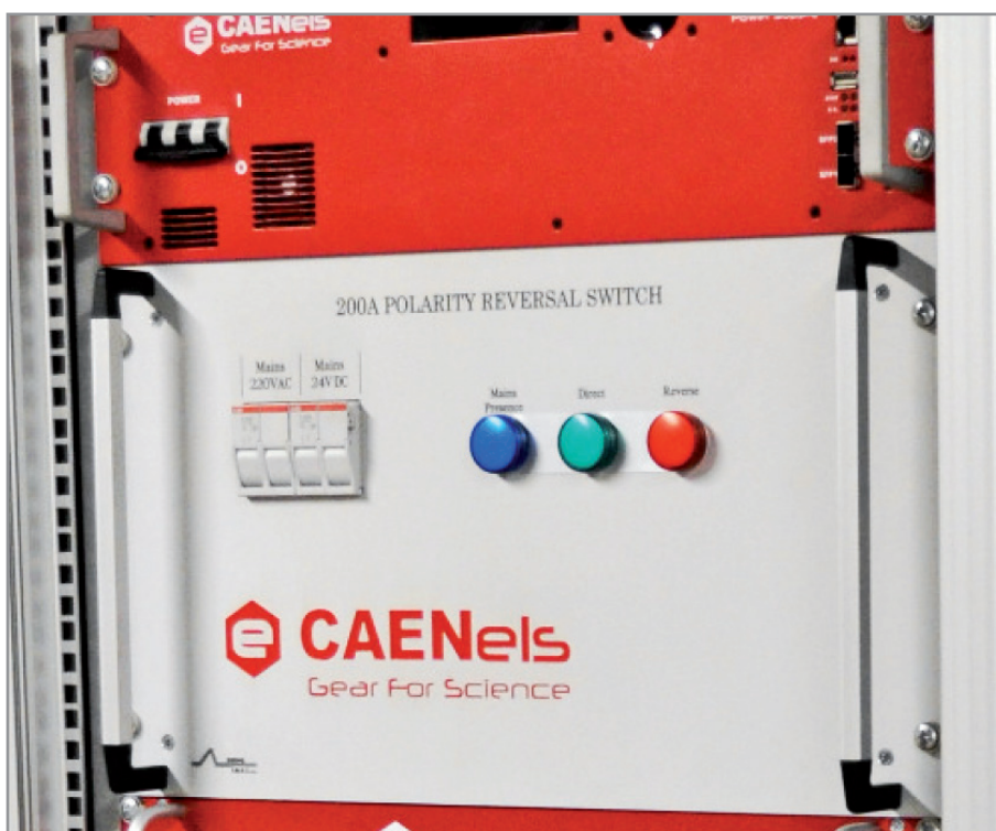
Installation of the Polarity Inverter with an NUPS unit
