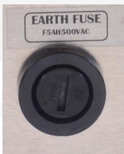
Figure 12: Earth fuse holder
