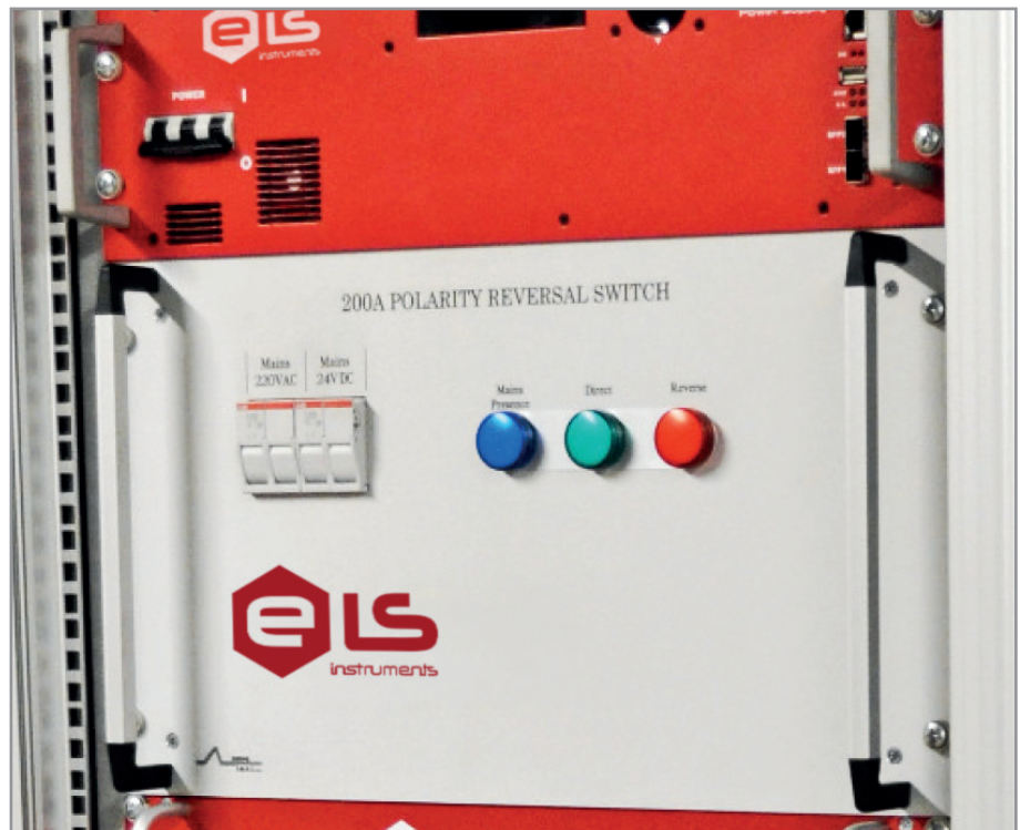
Installation of the Polarity Inverter with an NCPS unit
